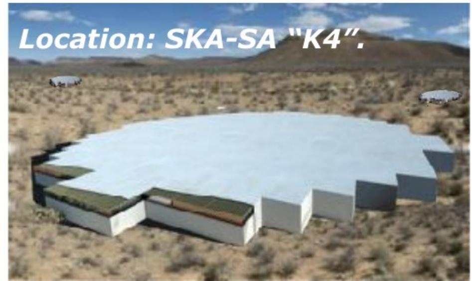
0.45-1.45GHz,  $A \sim 1500-2500 \text{m}^2$ , SEFD  $\sim 74-44 \text{Jy}$
